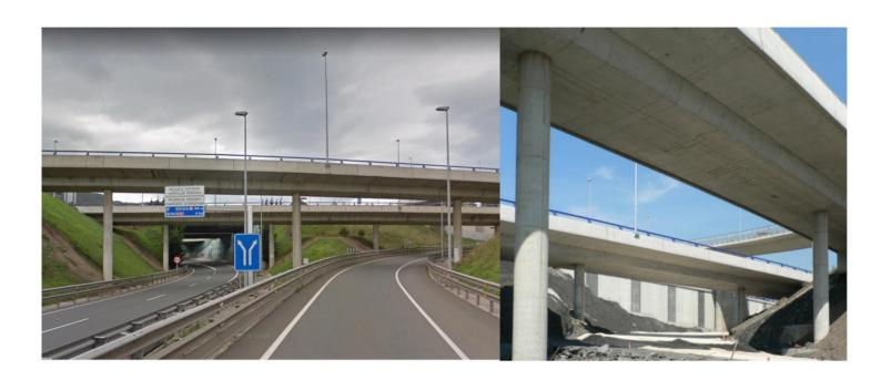
The reinforced hollow slabs cover a maximum span of 23.0m with maximum depths of 1.15m (L/20) and have been projected as bridges free of supports or expansion joints which therefore greatly reduce the maintenance costs. To do this, the circular shafts are embedded in the deck and the load beams and are founded on micro-piles.
